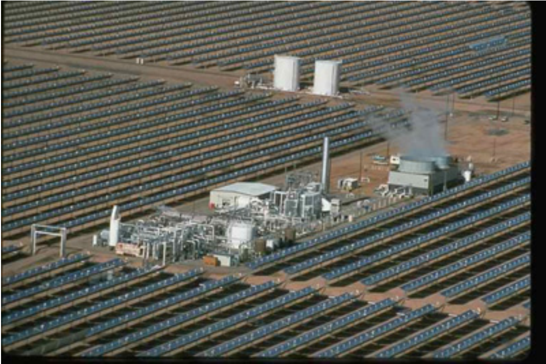
Figure 2: Photograph of the “parabolic trough” solar electricity generating systems (SEGS) in California, constructed in 1990. The parabolic trough collectors are traced to follow the sun from sunrise to sunset. The steam power plant is in the middle of the collector field. In the Gaza Solar Water&Power Source there would be desalination plants instead of cooling towers.
